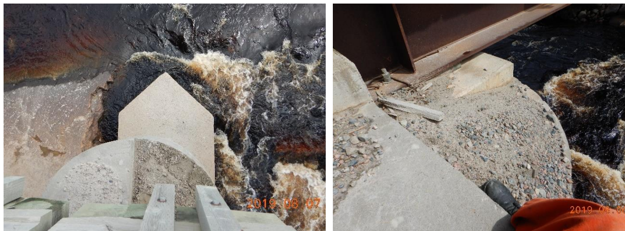
Figure 27 : Pile's bearing seat
