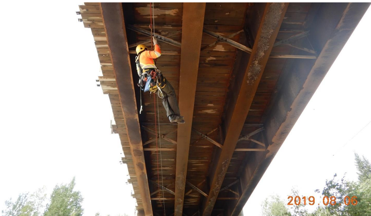
Figure 4 : Beams and wood deck
