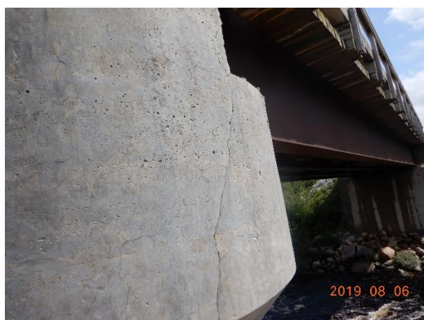
Vertical crack width < 0.8 mm
