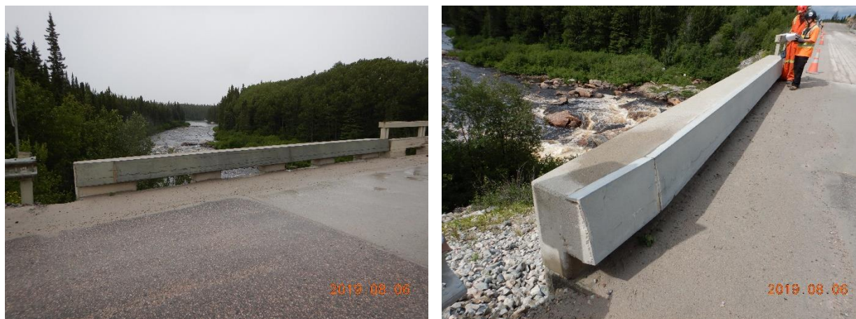
Figure 15 : Concrete guardrails
