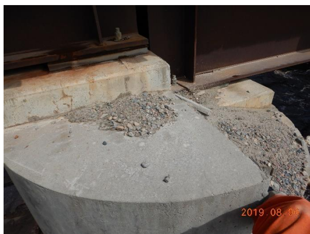
Vertical crack width < 0.8 mm
