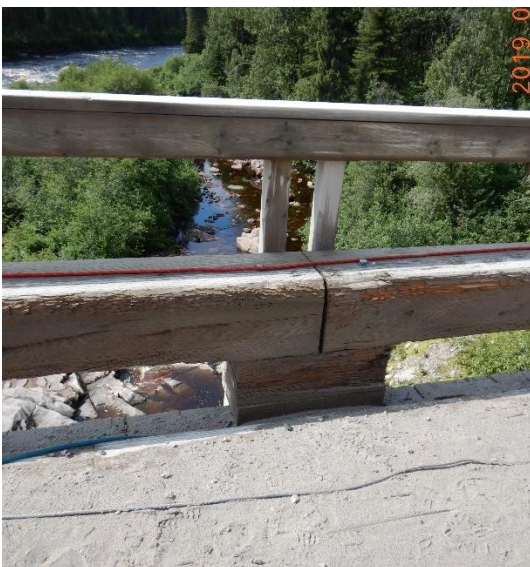
Typical curb and guardrails detail
