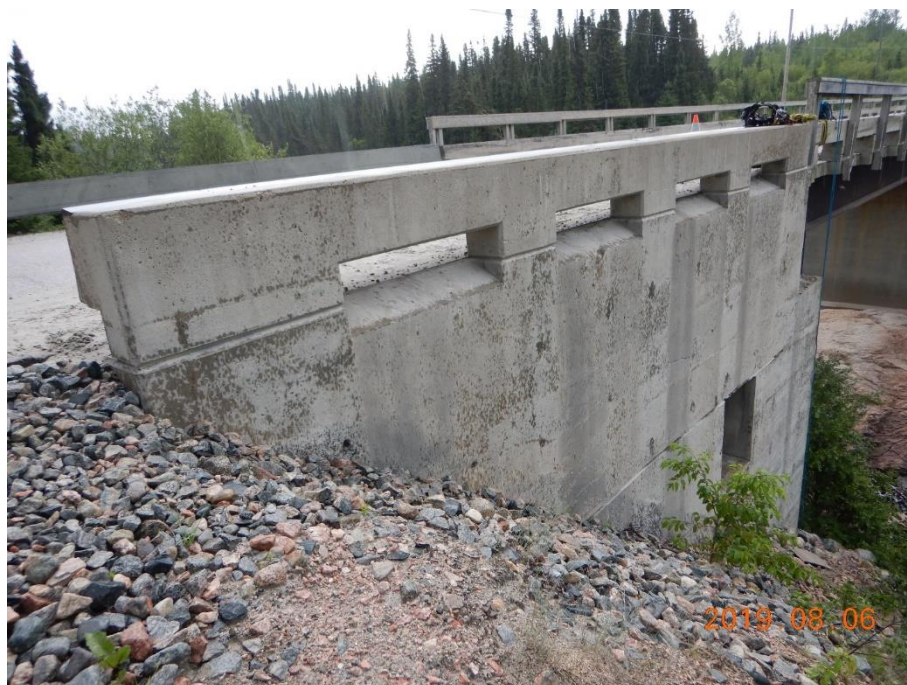
Figure 13 : Slope protection, wingwall no.1
