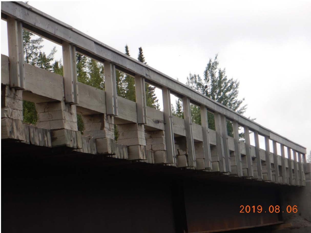
Figure 35 : Wood guardrails – span 2
