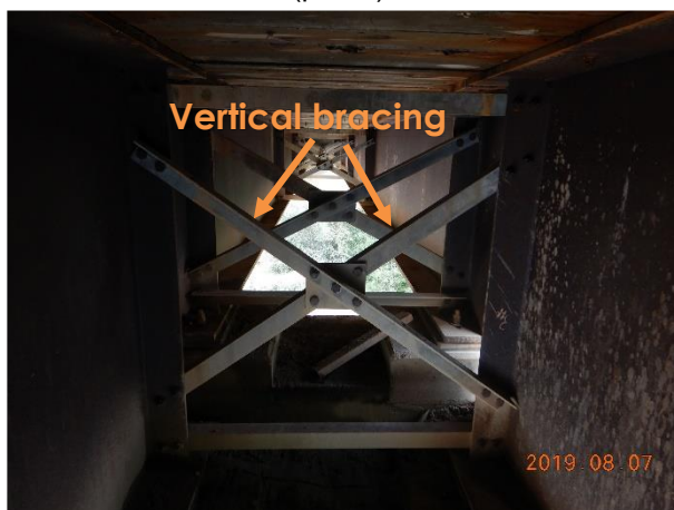
Span 1 – End vertical transverse bracings (pier 2)
