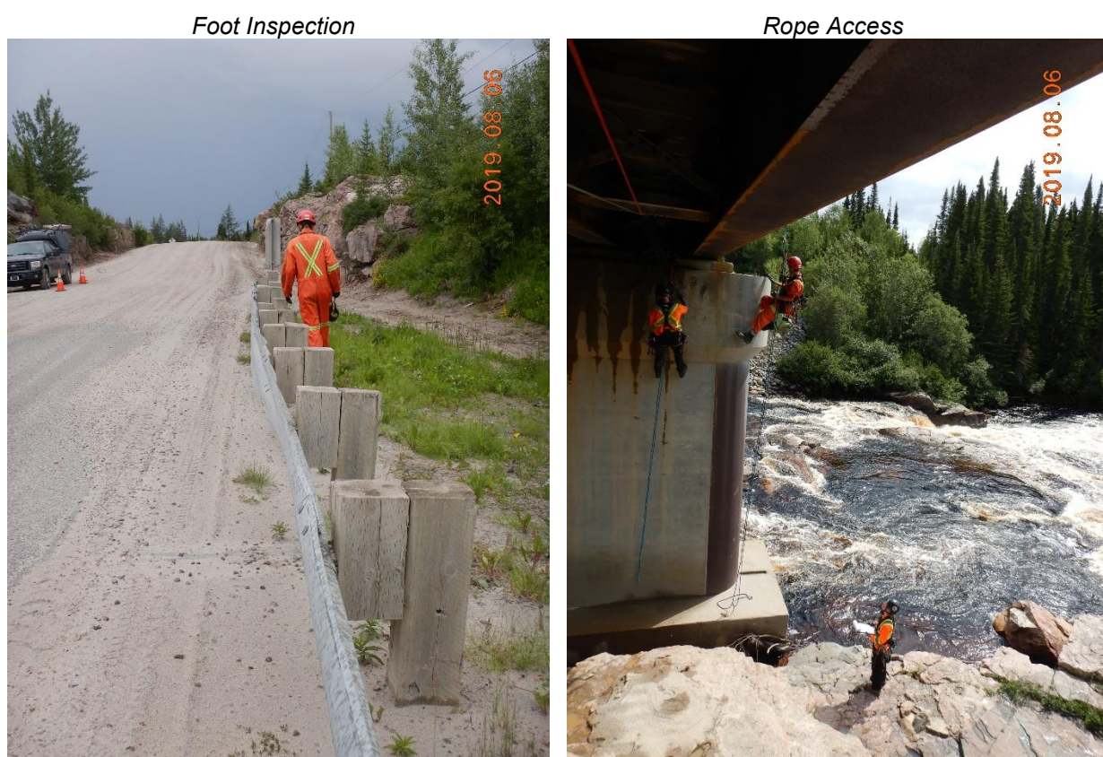
Figure 7 : Foot and Rope Access Inspection
