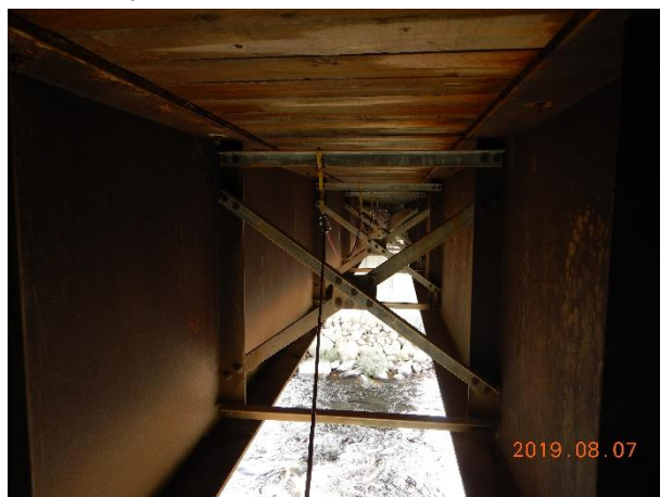
Span 2 – Timbers between beams
