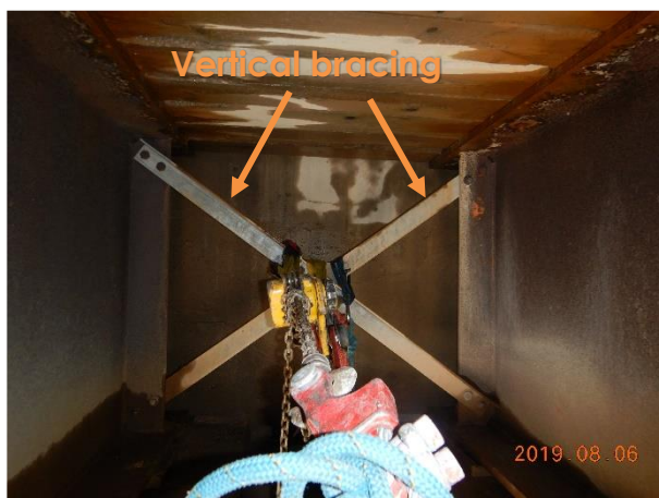
Span 1 – End vertical transverse bracings (pier 2)
