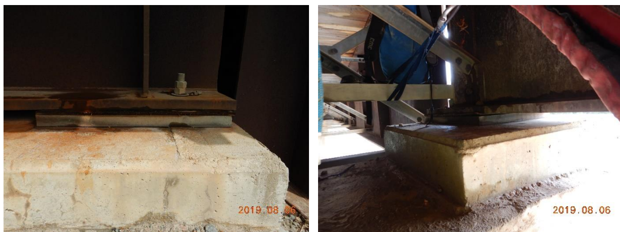
Figure 28 : Pile's bearings and pedestals
