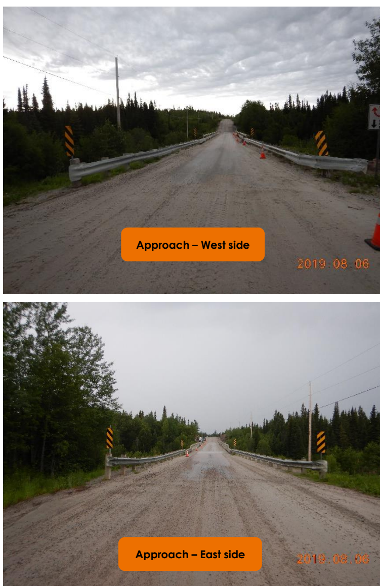
Figure 14 : Wood and galvanized steel Guardrails
