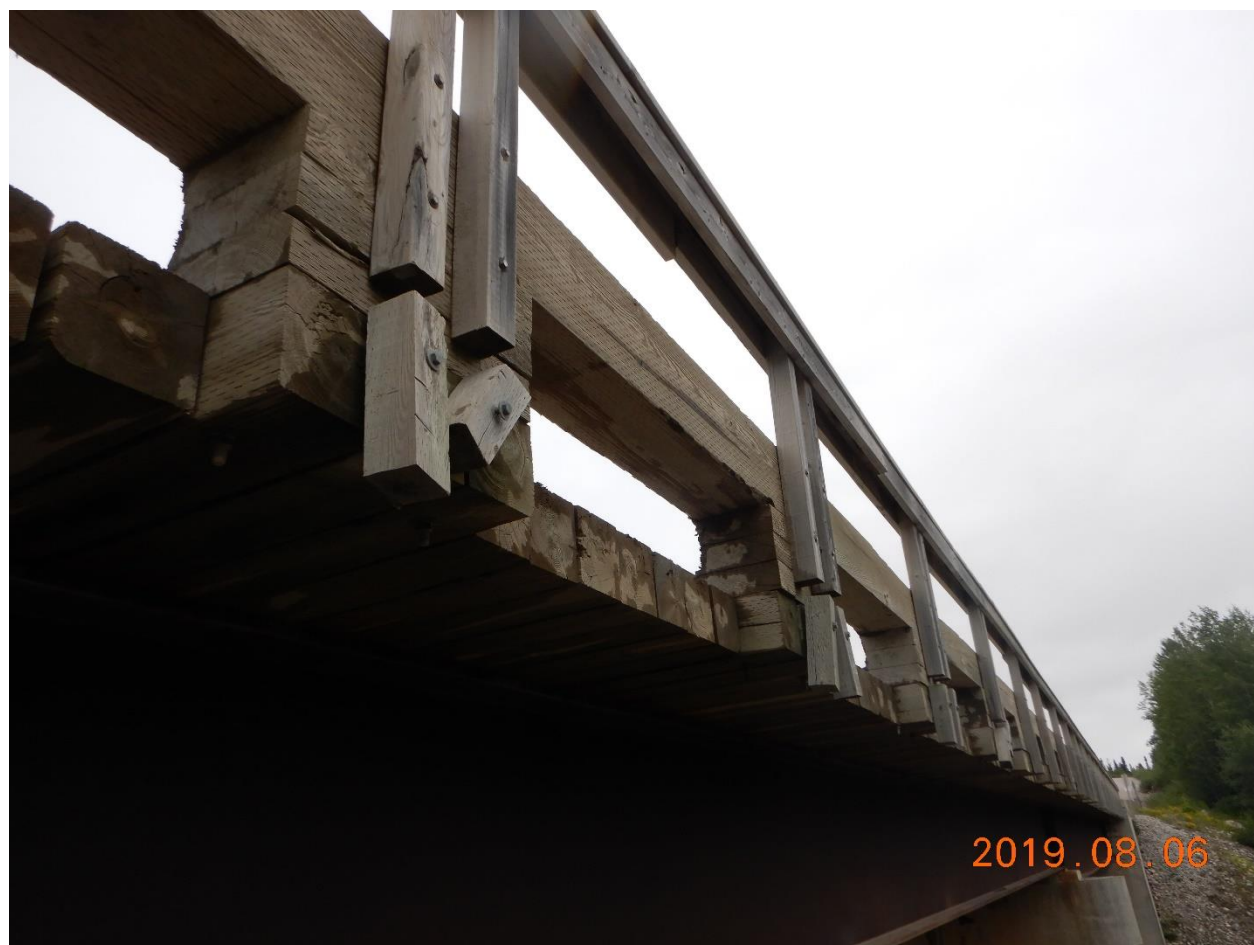
Figure 34 : Wood guardrails – span 1
