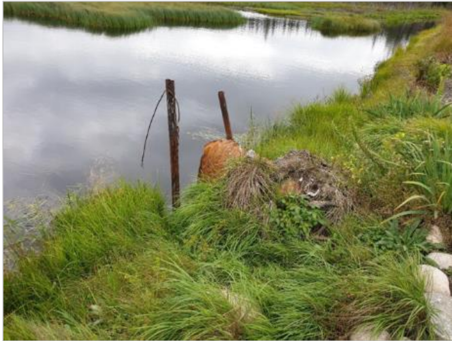
Figure 8.5-91: Existing 600mm Diameter CSP Culvert Crossing Grevet-Chapais Roadbed at KP 132.0. (The culvert is rusted but seems functional)
