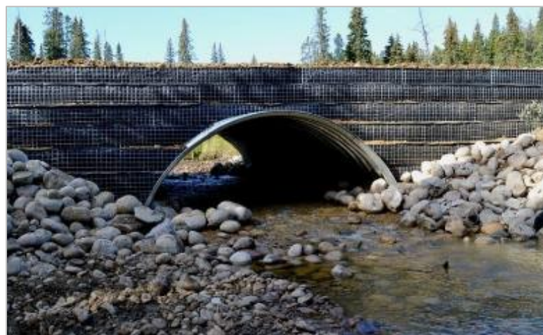
Figure 8.5-89: Example of a Bottomless Structural Steel Plate Arch Culvert
