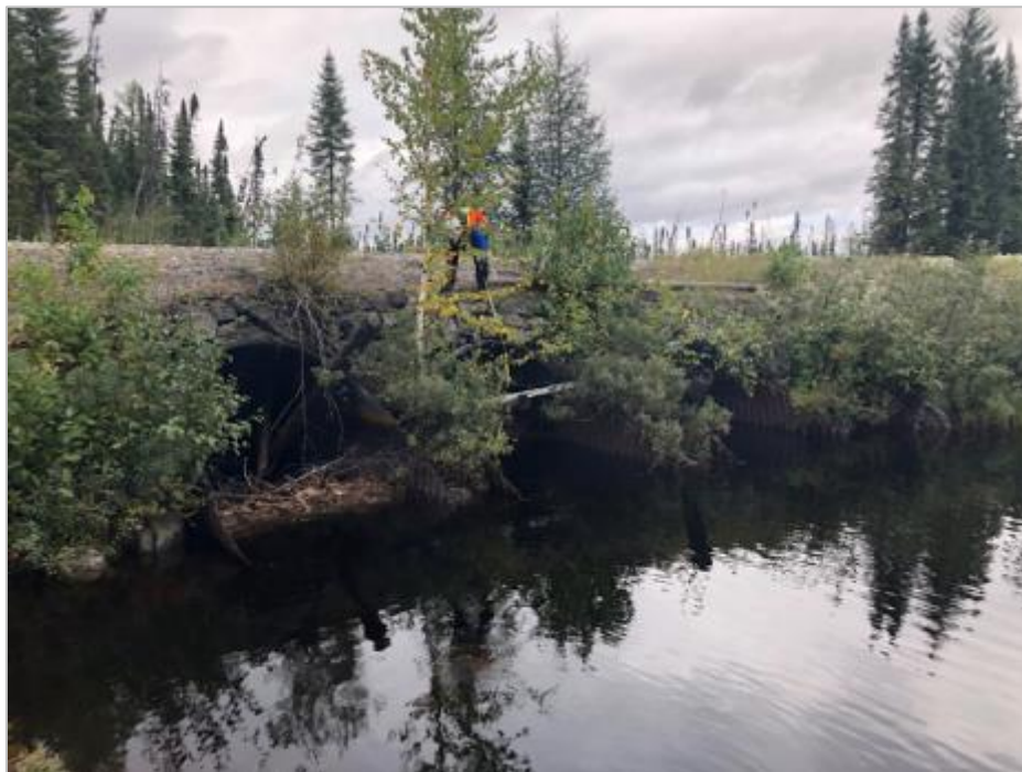
Figure 8.5-94: Existing 3 x 2400mm CSP Culverts Crossing Grevet-Chapais Roadbed at KP 229.2
