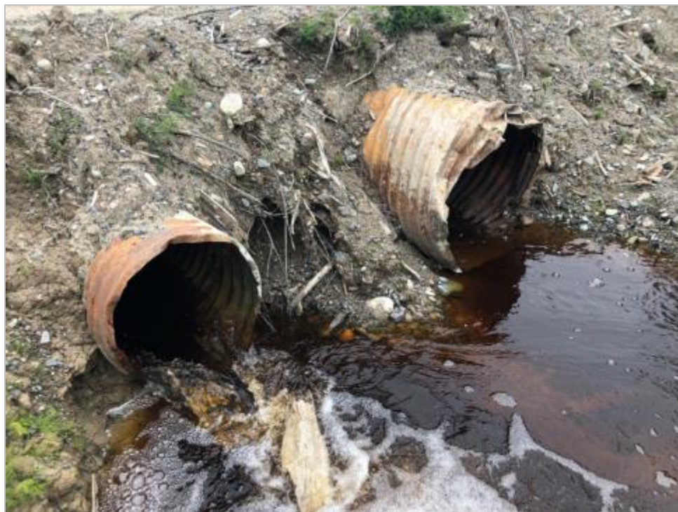
Figure 8.5-92: Existing 1000mmØ and 600mmØ CSP Culverts Crossing Grevet-Chapais Roadbed at KP 164.1. (The culverts are rusted and slightly dented but seem functional)
