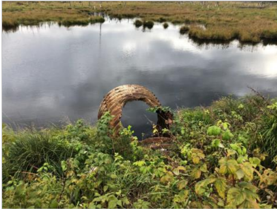
Figure 8.5-93: Existing \pm 1500\text{mm}\varnothing CSP Culvert Crossing Grevet-Chapais Roadbed at KP 220.1. (The culvert is rusted and broken)
