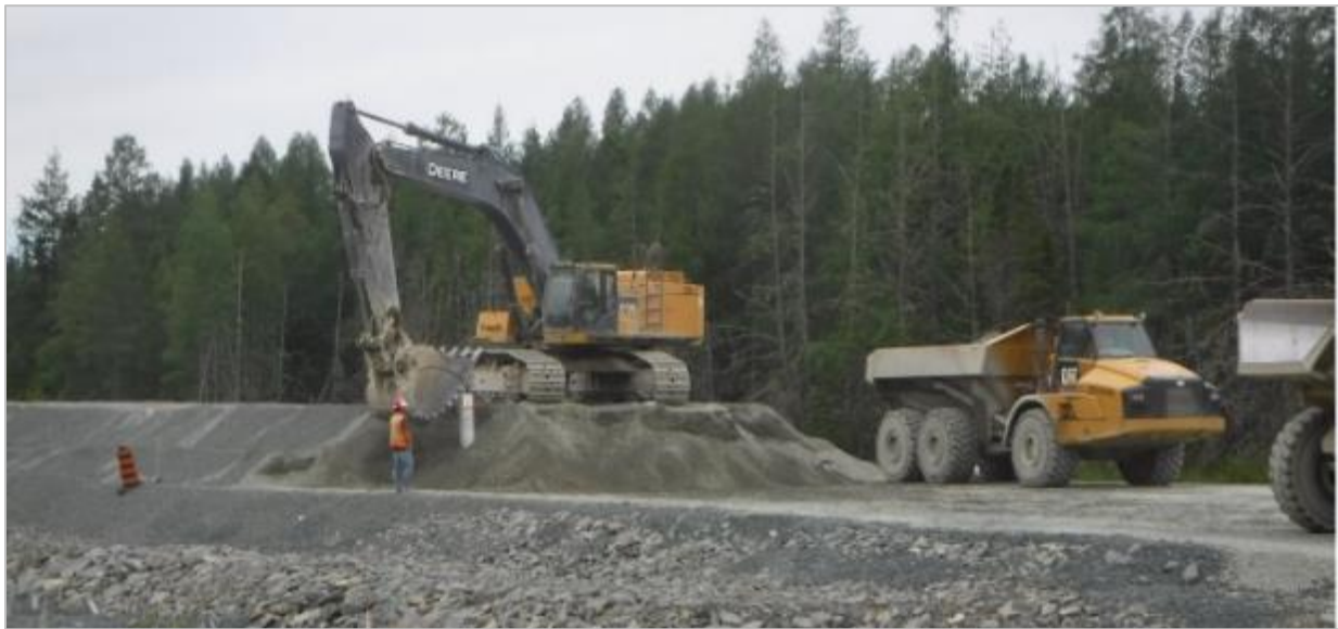
Figure 8.5-23 : Removal of Granular Surcharge Material – Manual on Compressible Soils
