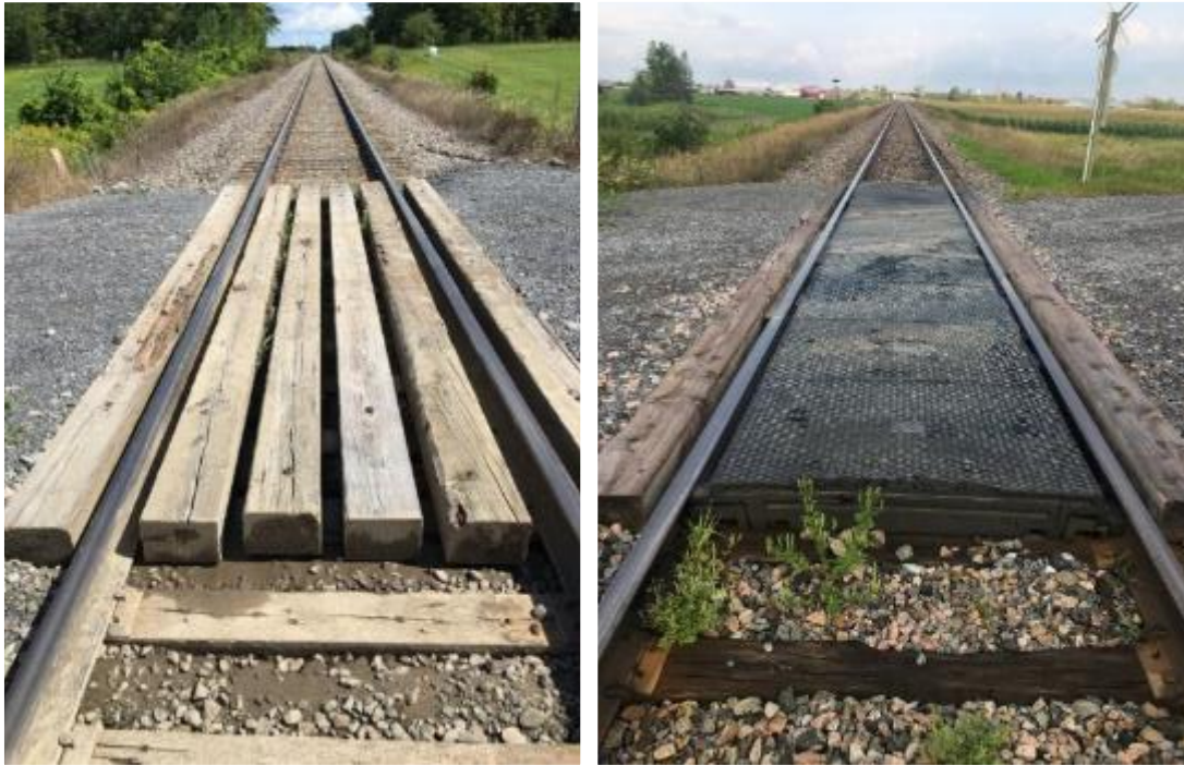
Figure 8.5-36: Two Examples of Minor Level Crossings. On the left, a level crossing with wood plank-based surface. On the right, a level crossing with a rubber-pad surface.
