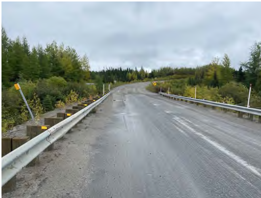
Photo : 22 | On the bridge
