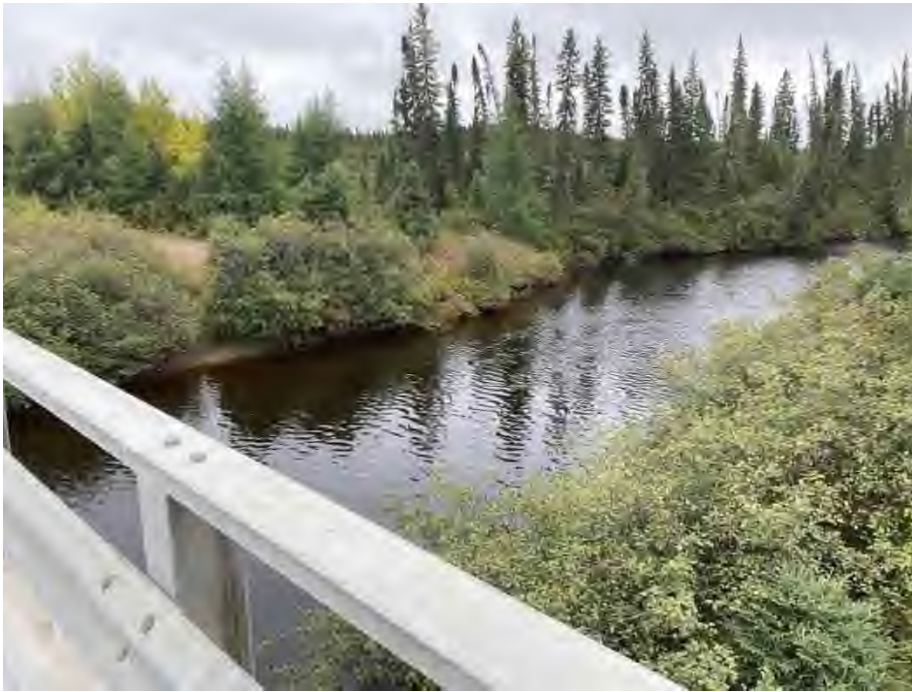
Photo : 15 Bridge looking at downstream
