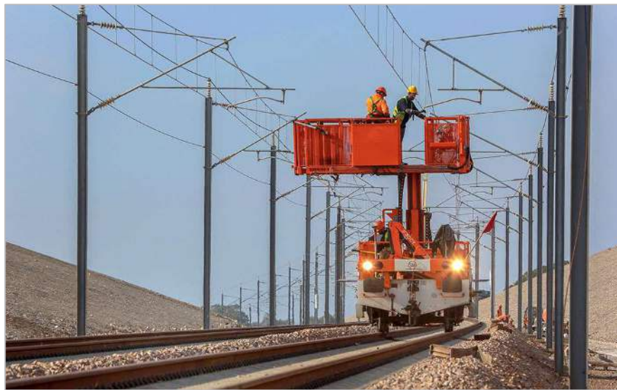
Figure 4-2: OCS 2*25 kVac type for main tracks
