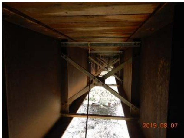
Span 2 – Timbers between beams
