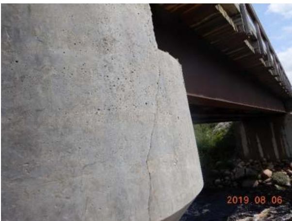
Vertical crack width < 0.8 mm
