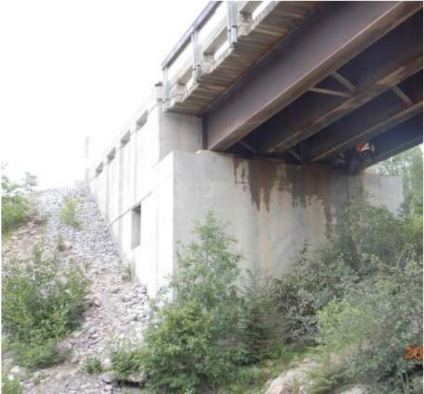
West abutment / Axis 1
