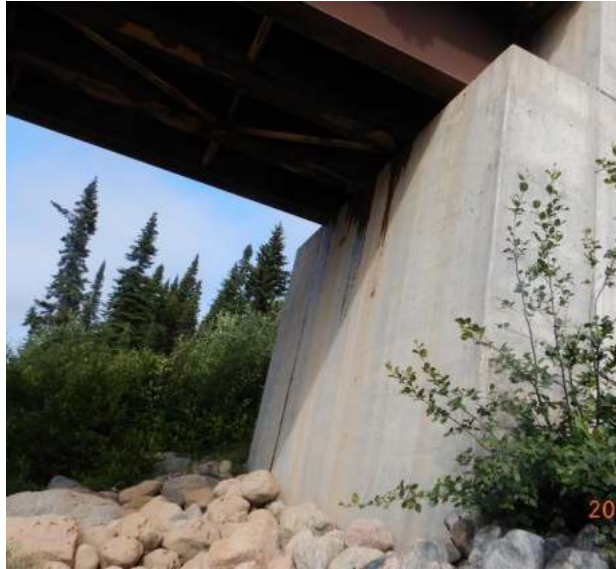
East abutment / Axis 3
