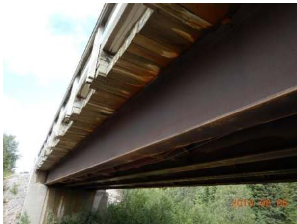
Span 1 – Timbers' extremity
