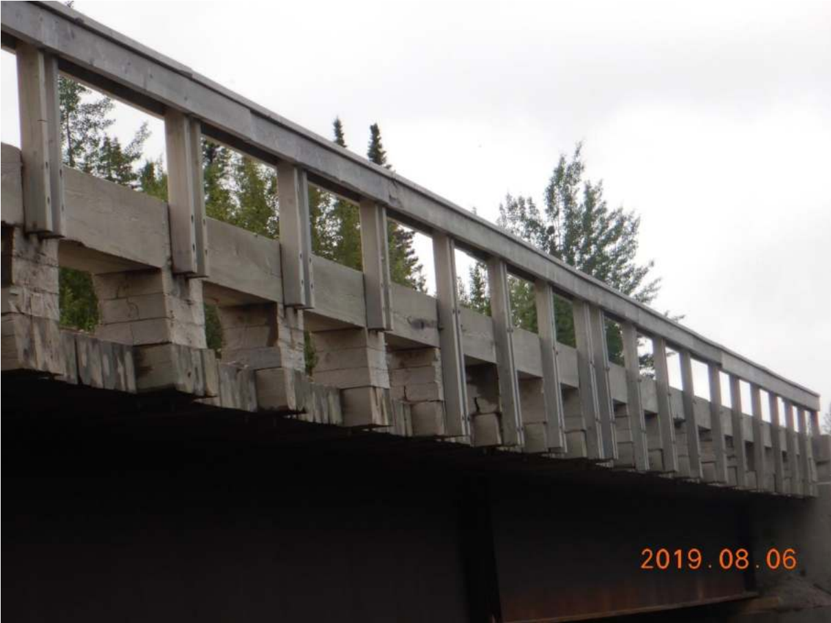
Figure 35 : Wood guardrails – span 2
