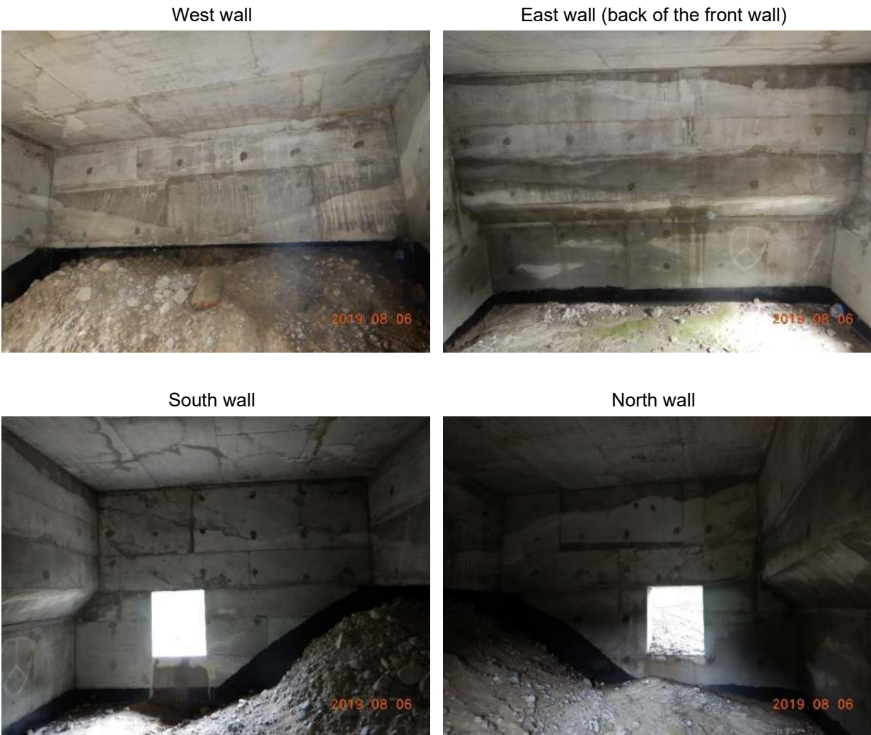
Figure 22 : West abutment's interior
