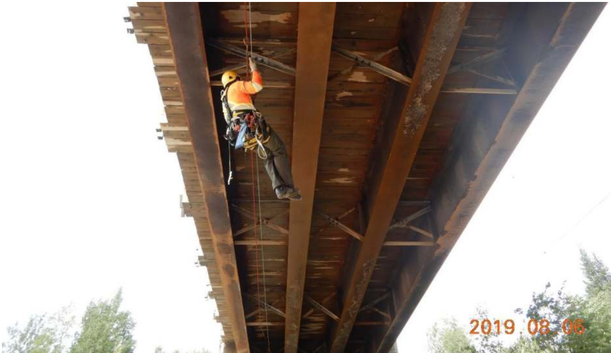
Figure 4 : Beams and wood deck
