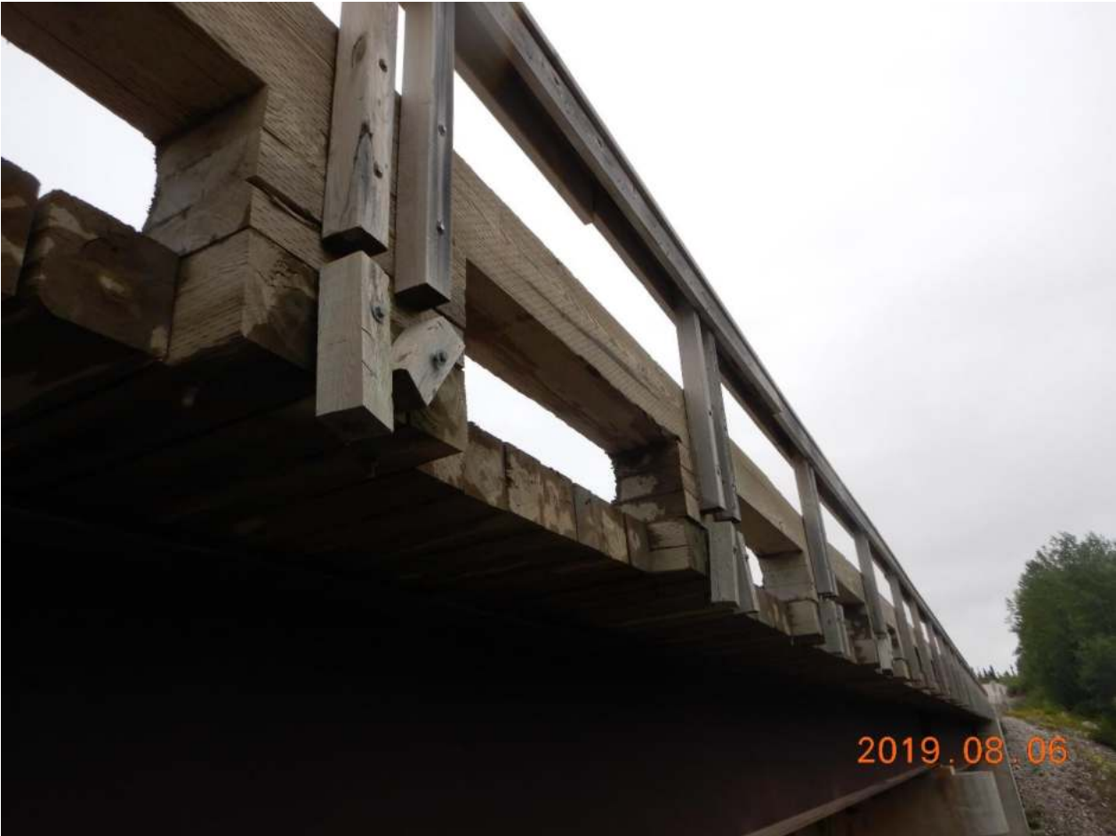
Figure 34 : Wood guardrails – span 1
