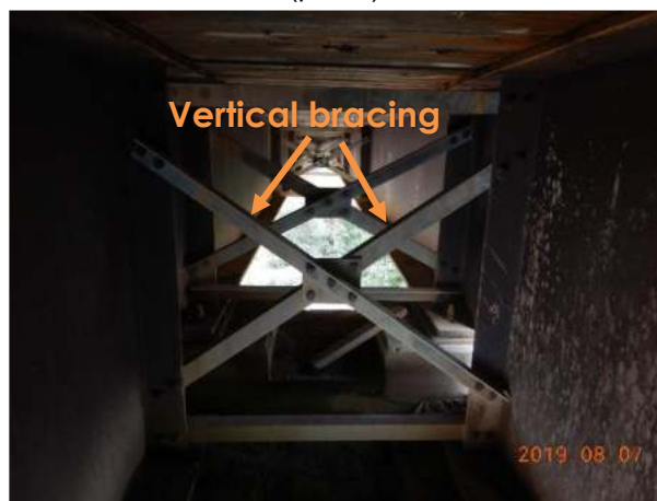
Span 1 – End vertical transverse bracings (pier 2)
