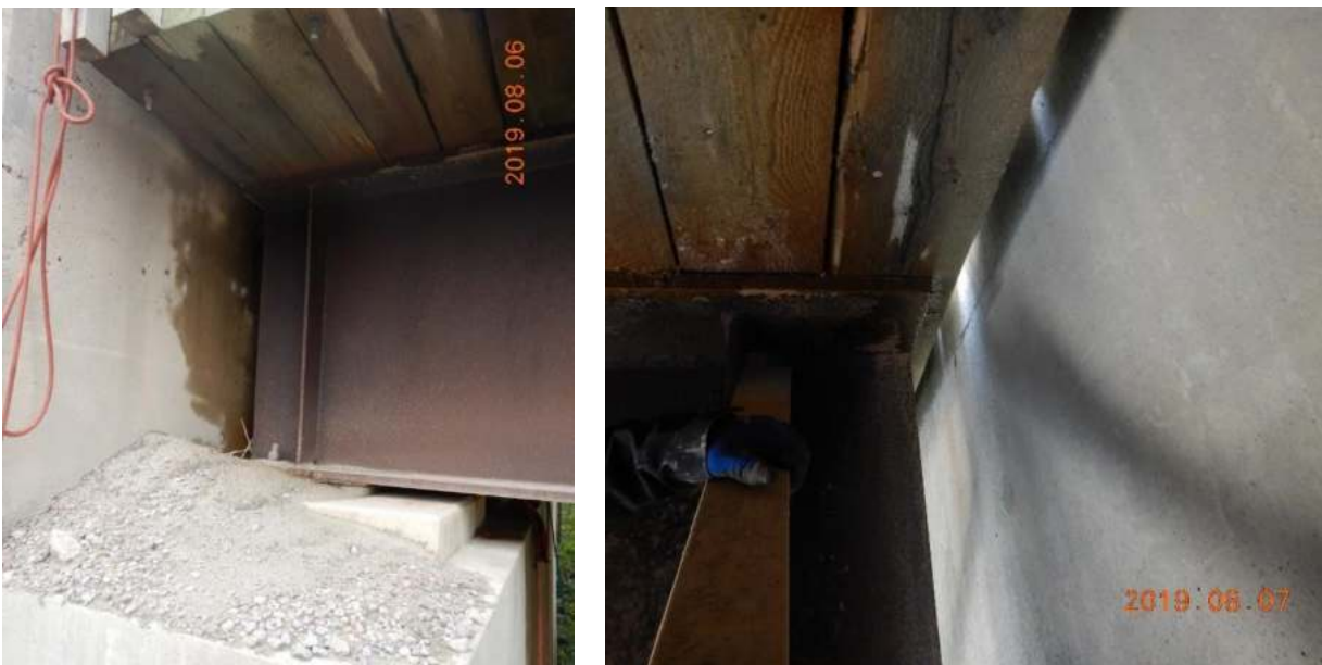
Figure 21 : Ballast walls (Left: West and Right: East)
