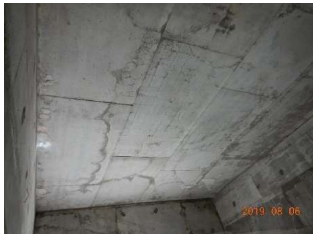
West abutment: Deck soffit
