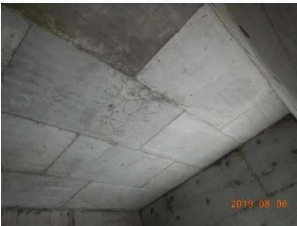
East abutment: Deck soffit
