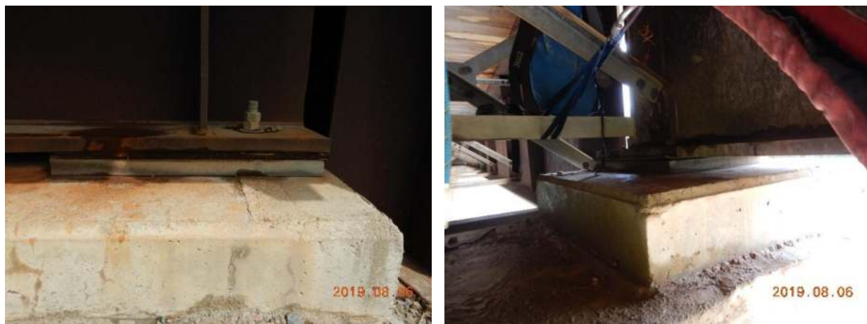
Figure 28 : Pile's bearings and pedestals
