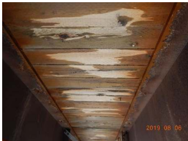
Span 1 – Timbers between beams
