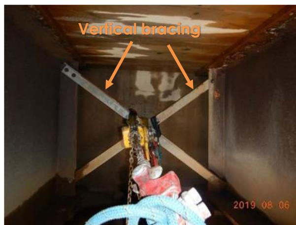
Span 1 – End vertical transverse bracings (pier 2)
