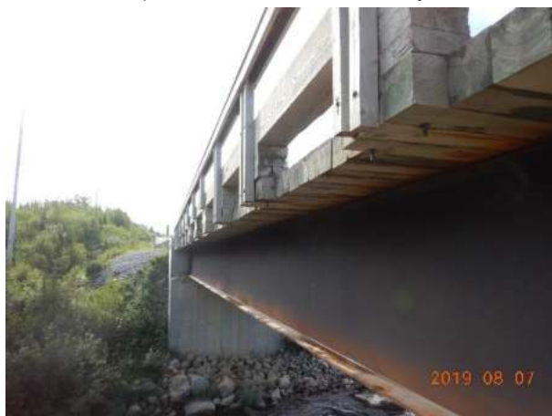
Span 2 – Timbers' extremity
