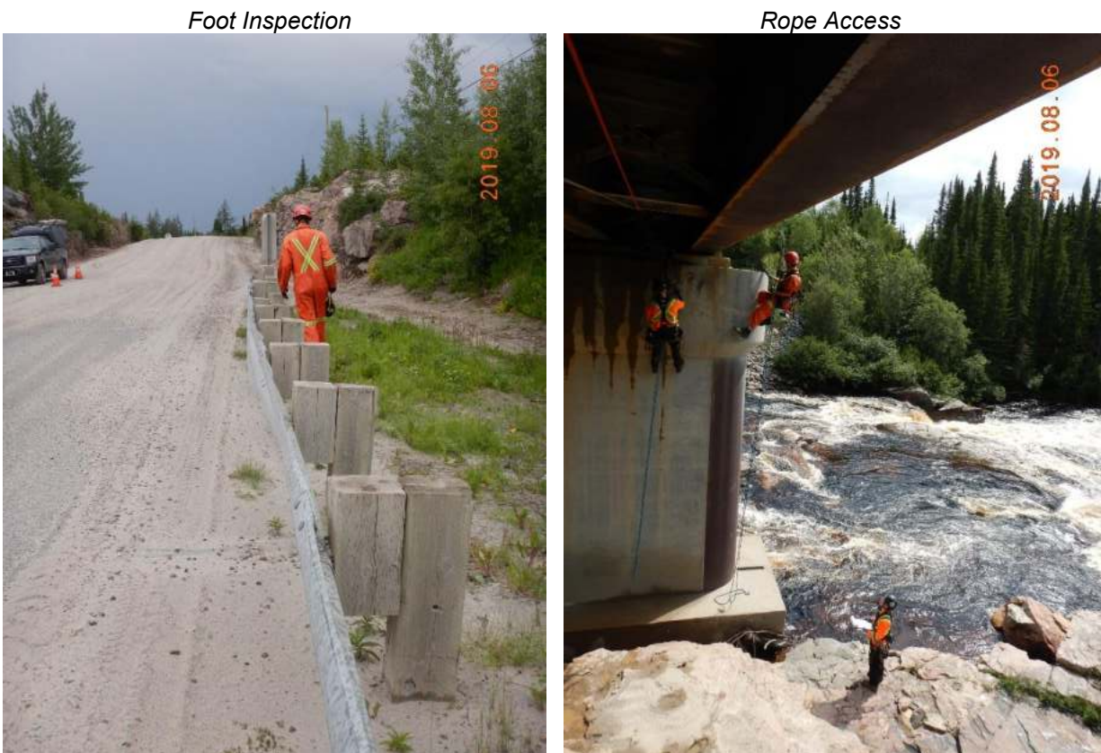
Figure 7 : Foot and Rope Access Inspection
