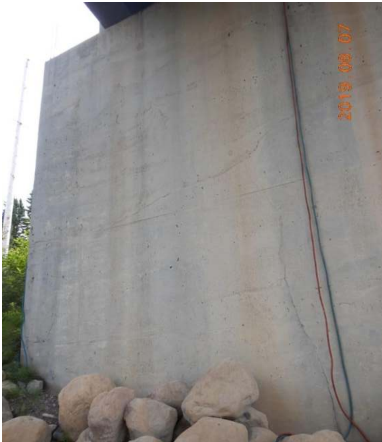
Figure 18 : Cold joint and narrow cracks on the West front wall
