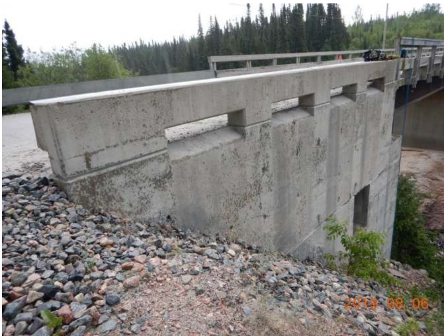
Figure 13 : Slope protection, wingwall no.1
