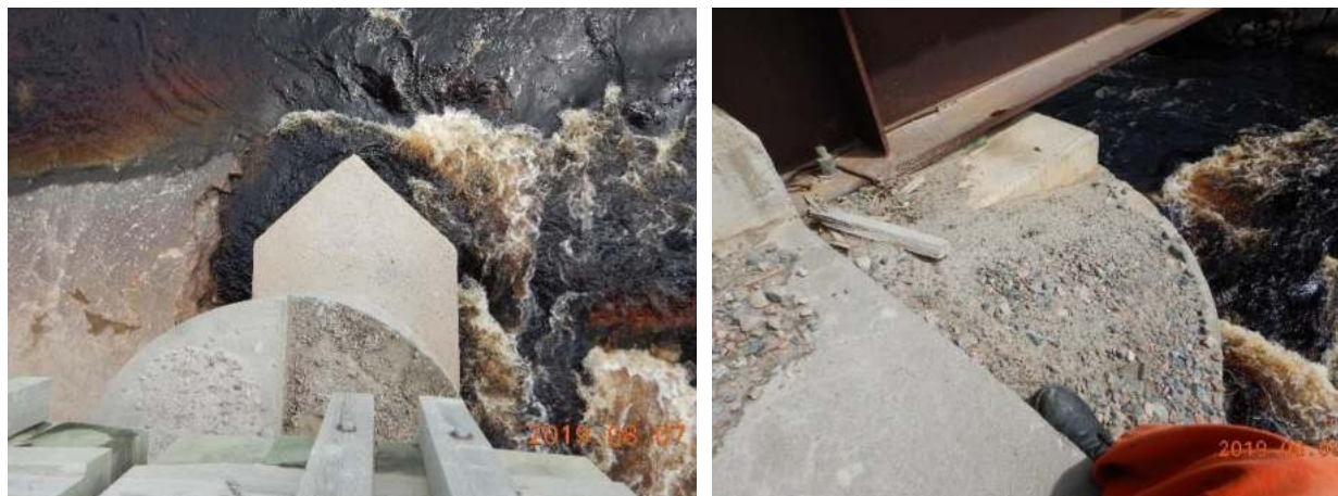
Figure 27 : Pile's bearing seat
