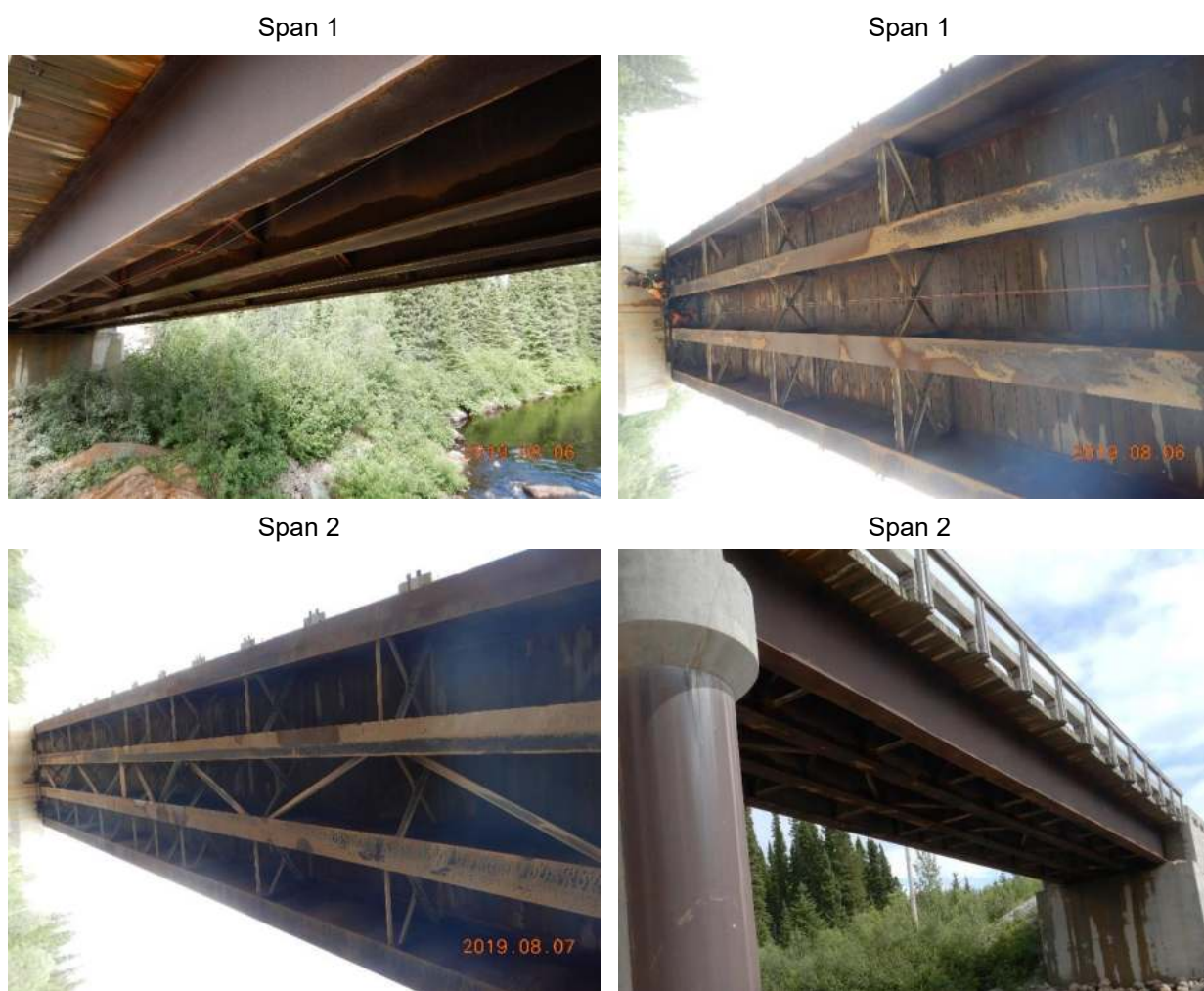
Figure 29 : Beams general views
