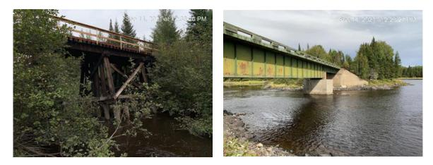
Figure 3-3: Timber Trestle Bridge at MP 105.6 (Left) and DPG' Steel Bridge at MP 122.3(Right).
