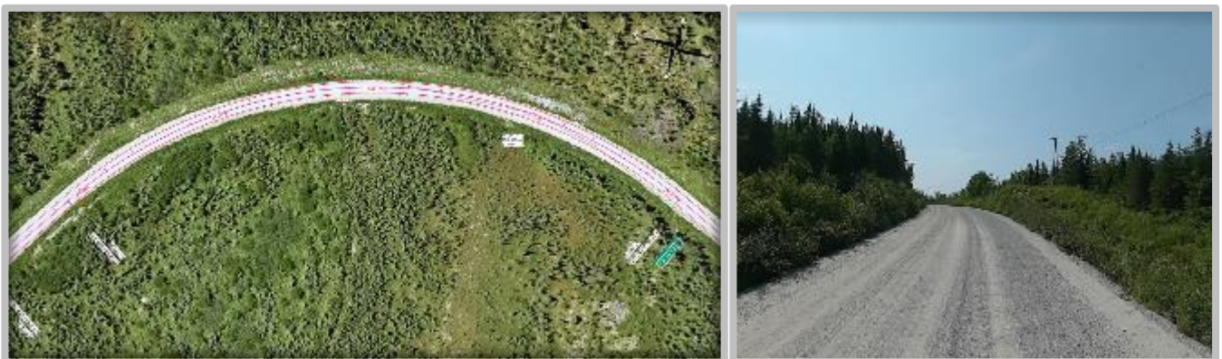
Figure 8.7-3 : Street View July 2022 - Curve at kilometer 242 (Route du Nord)
