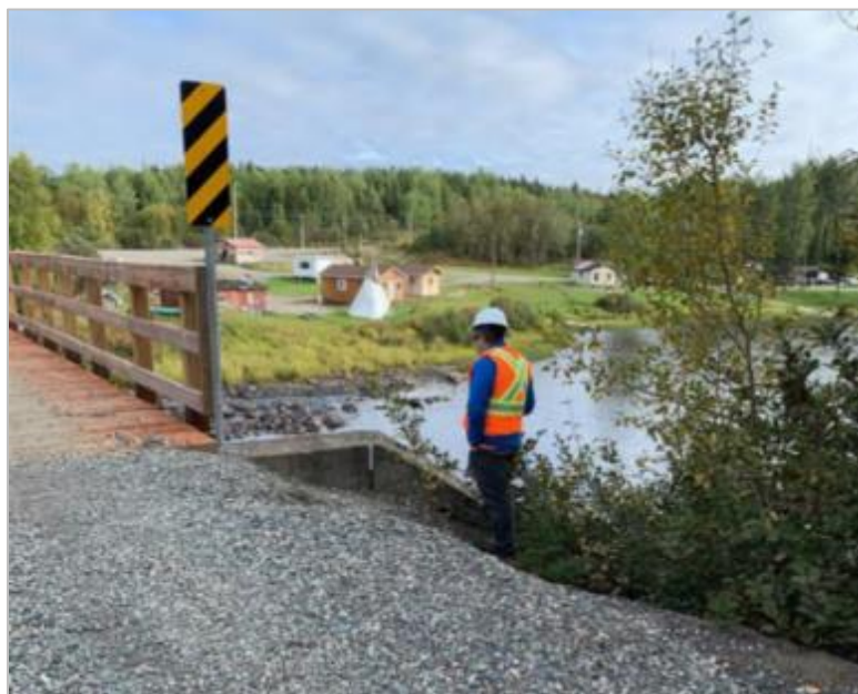
Figure 8.5-71: Inspection of O'Sullivan River Bridge
