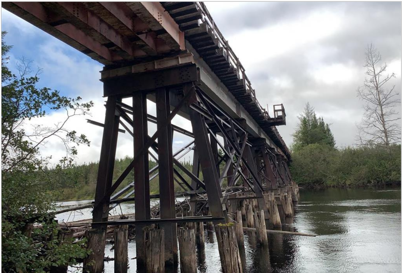
Figure 8.5-80: General View of the Bridge at KP 156.00
