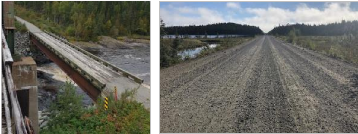
Figure 8.9-4: Bridge Site and Road Pictures by VEI
