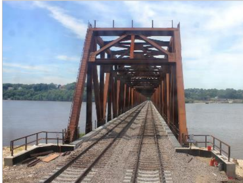
Figure 8.5-70: Example of TPG Bridge
