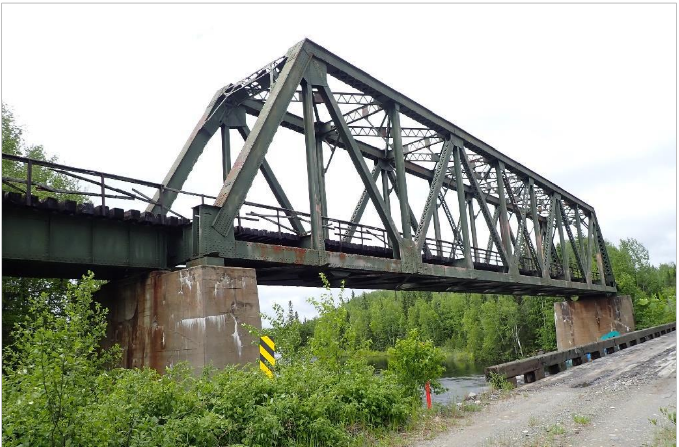
Figure 8.5-78: General View of the Bridge at KP 201.72
