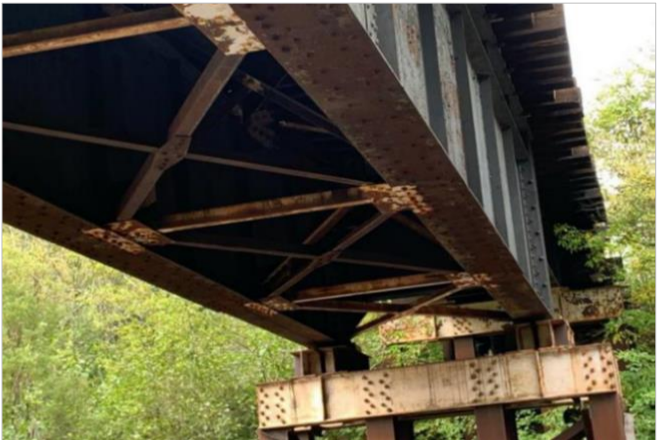
Figure 8.5-73: General View of the Bridge at KP 163.85
