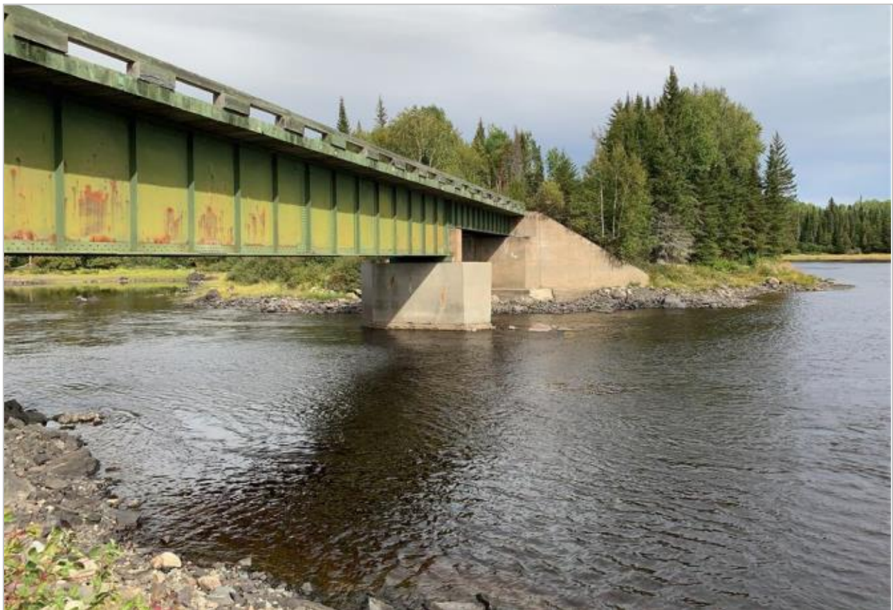
Figure 8.5-77: General View of the Bridge at KP 196.86
