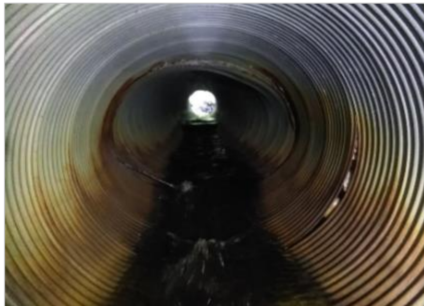
Figure 8.7-9: Inspected culverts on the Route du Nord
