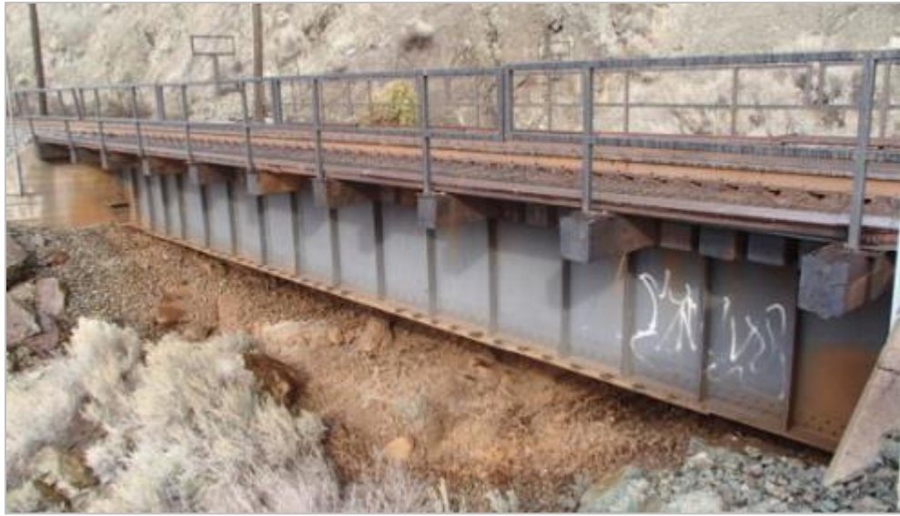
Figure 8.5-68: Example of DPG Bridge
