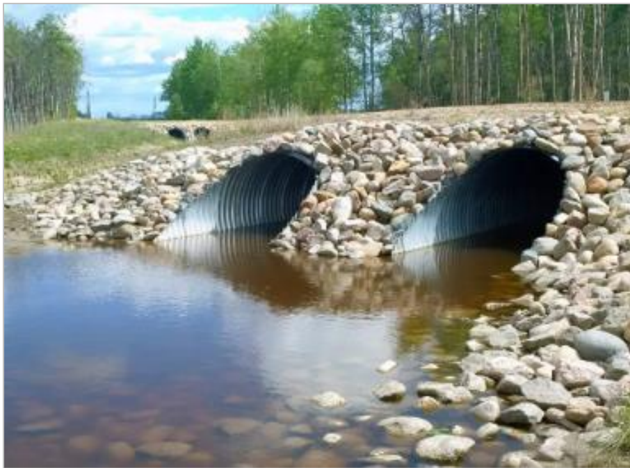
Figure 8.5-96: Example of a CSP Culvert
