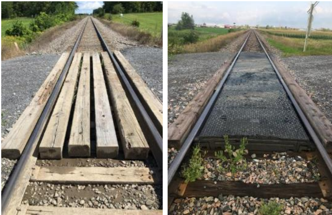
Figure 8.5-40: Two Examples of Minor Level Crossings
