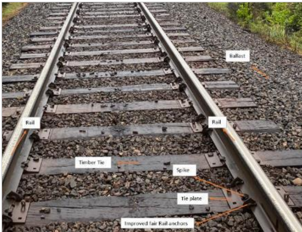
Figure 8.5-29: Track Structure Components
