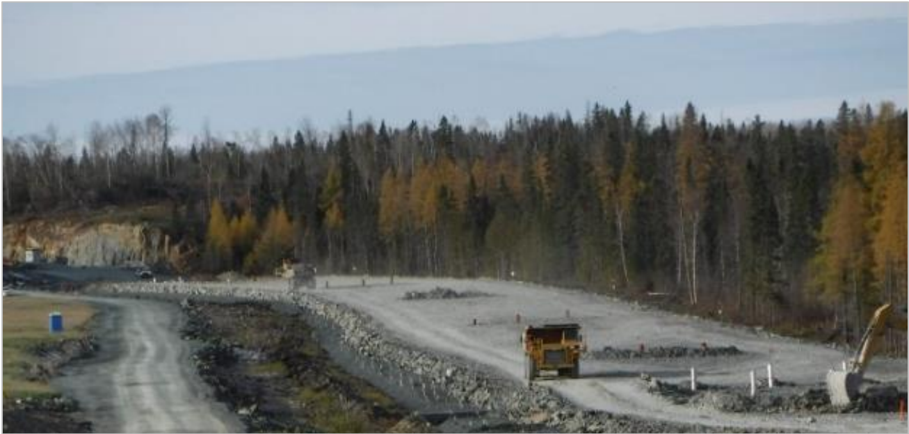
Figure 8.5-23: Fill Placement During Embankment Construction
