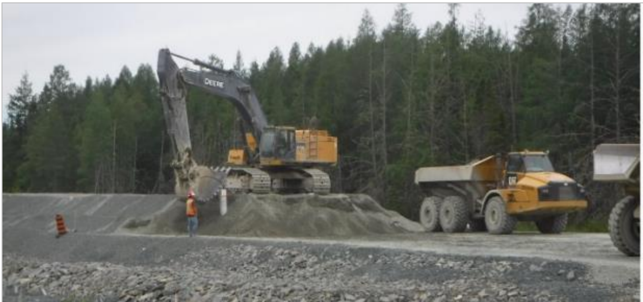
Figure 8.5-27: Removal of Granular Surcharge Material – Manual on Compressible Soils
