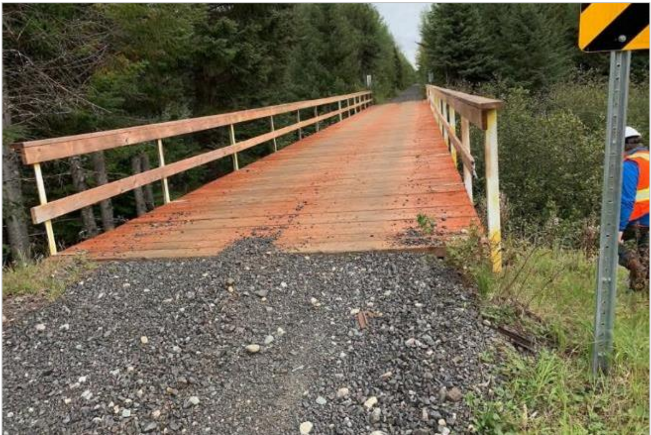
Figure 8.5-75: General View of the Bridge at KP 169.95
