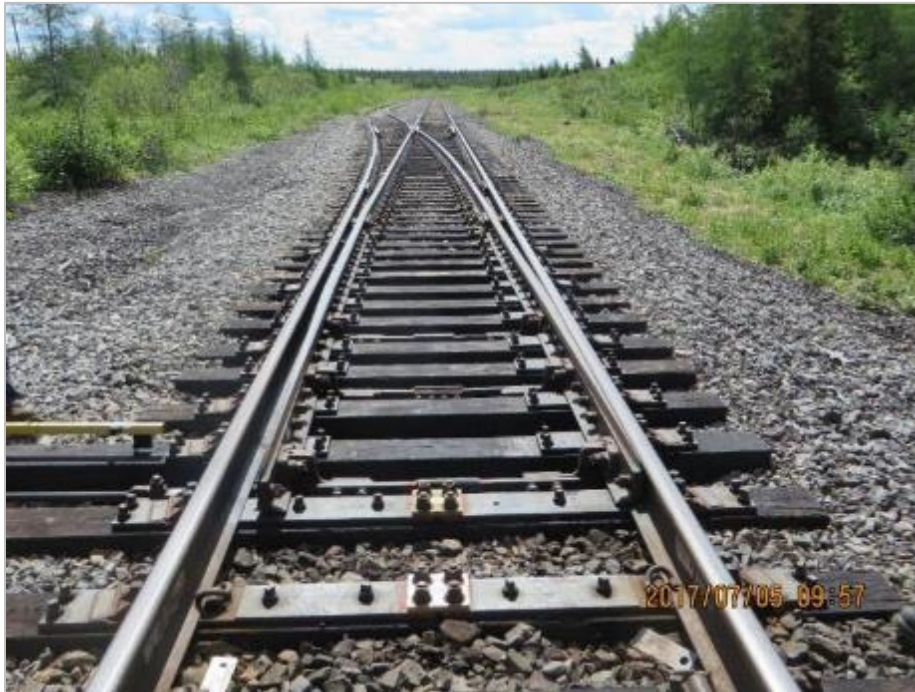
Figure 8.5-31: Picture of a Typical No. 8 Turnout
