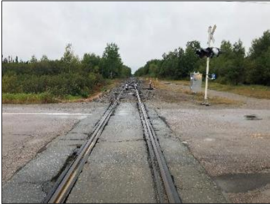
Figure 8.9-2: Crossing on Matagami Sub (25 mph Speed Limit)
