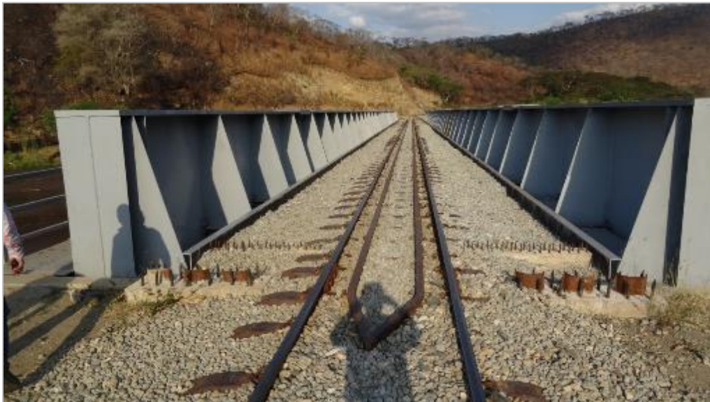
Figure 8.5-69: Example of TPG Bridge
