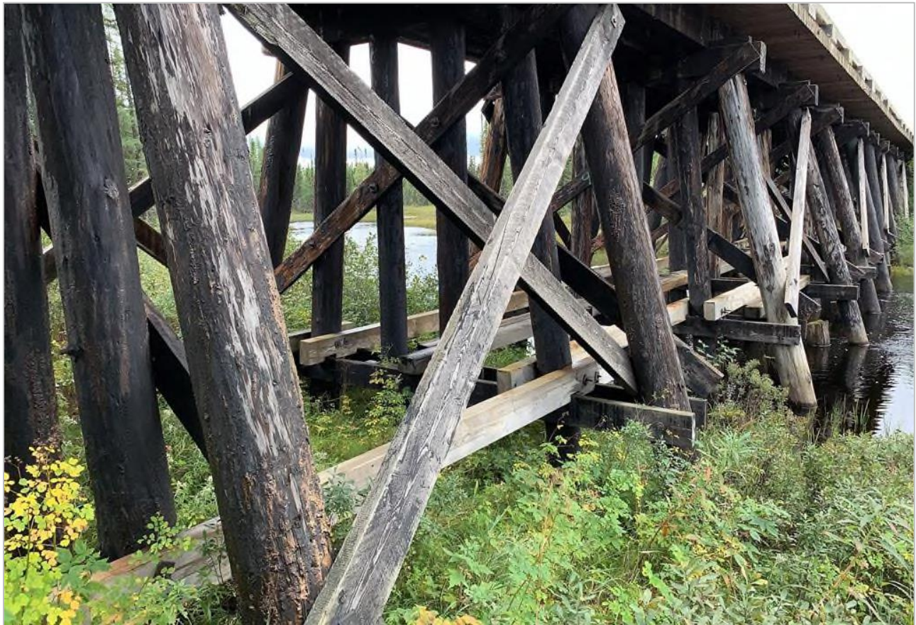
Figure 8.5-79: General View of the Bridge at KP 236.71
