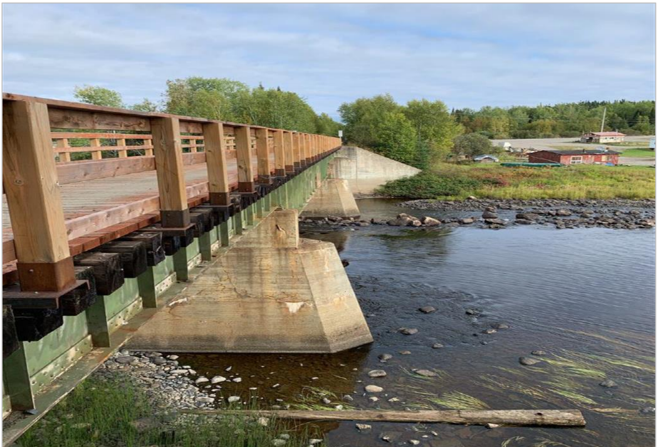
Figure 8.5-72: General View of the Bridge at KP 146.50
