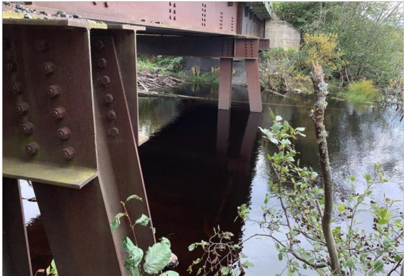
Figure 8.5-74: General View of the Bridge at KP 167.59
