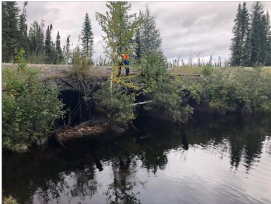
Figure 8.5-102: Existing 3 x 2400 mm CSP Culverts Crossing Grevet-Chapais Roadbed at KP 229.2
