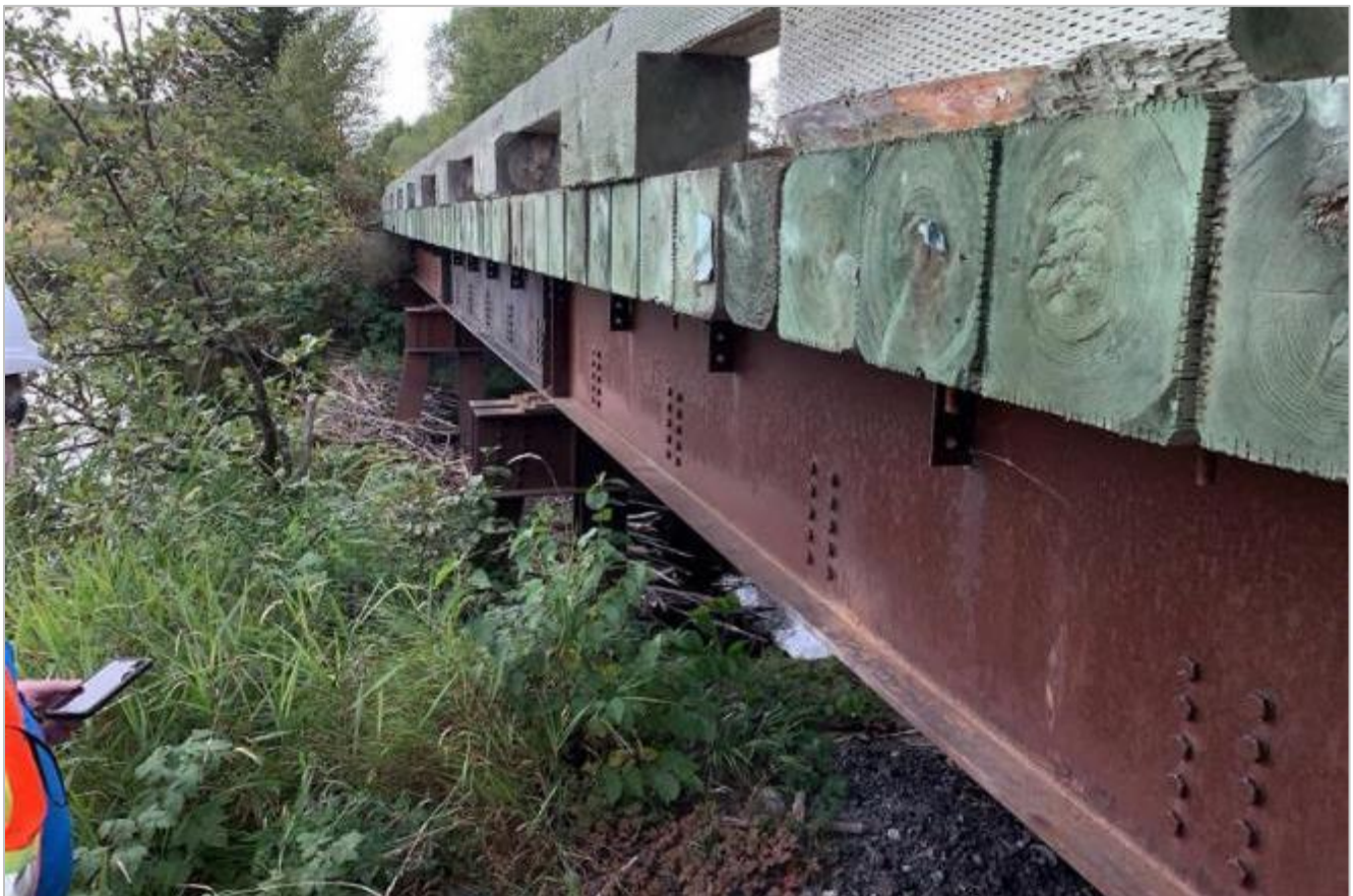
Figure 8.5-76: General View of the Bridge at KP 191.15
