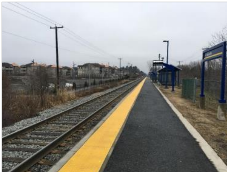
Figure 8.5-55: Example of a Passenger Station Platform
