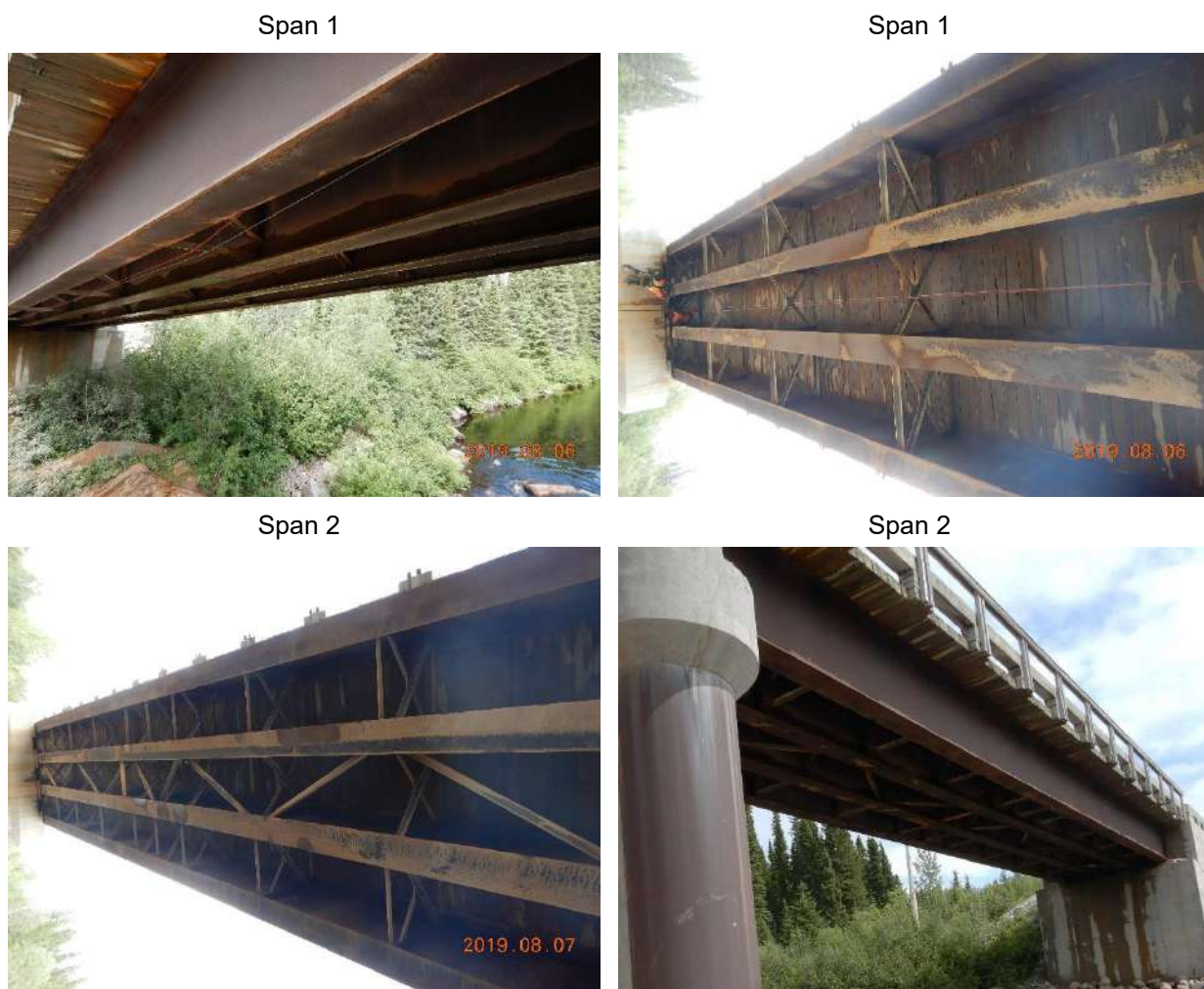
Figure 29 : Beams general views
