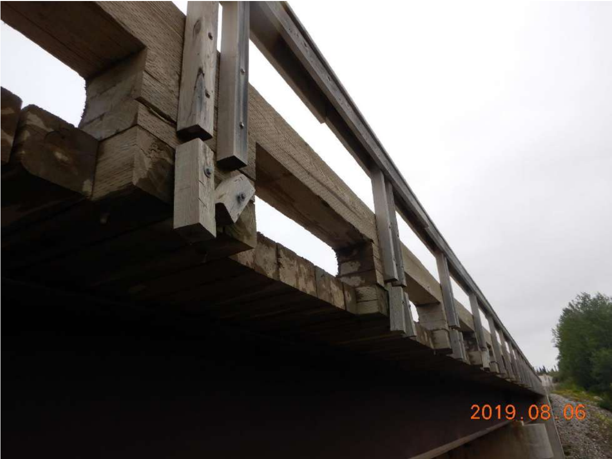
Figure 34 : Wood guardrails – span 1
