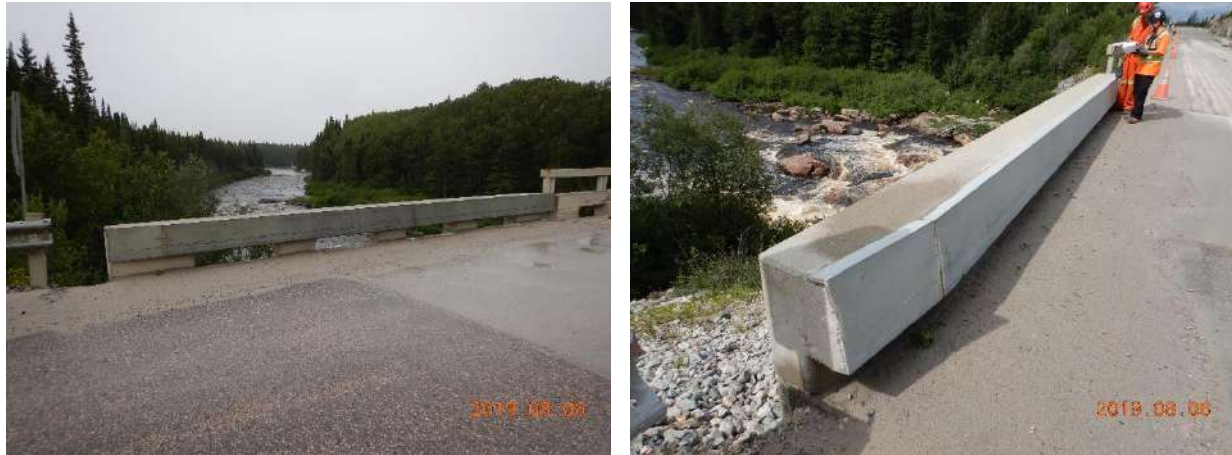
Figure 15 : Concrete guardrails
