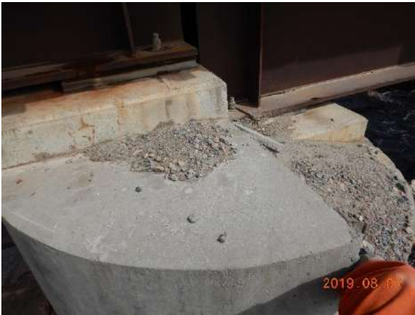
Vertical crack width < 0.8 mm
