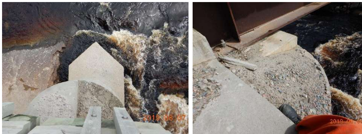
Figure 27 : Pile's bearing seat
