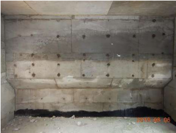
West wall (back of the front wall)
