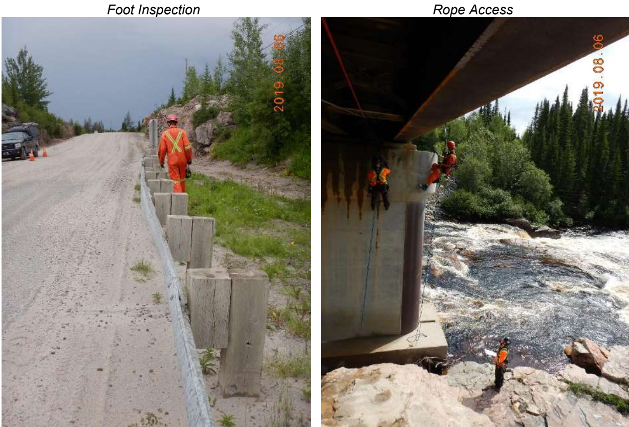
Figure 7 : Foot and Rope Access Inspection
