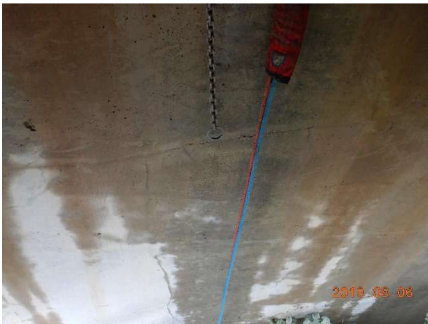
Figure 18 : Cold joint and narrow cracks on the West front wall
