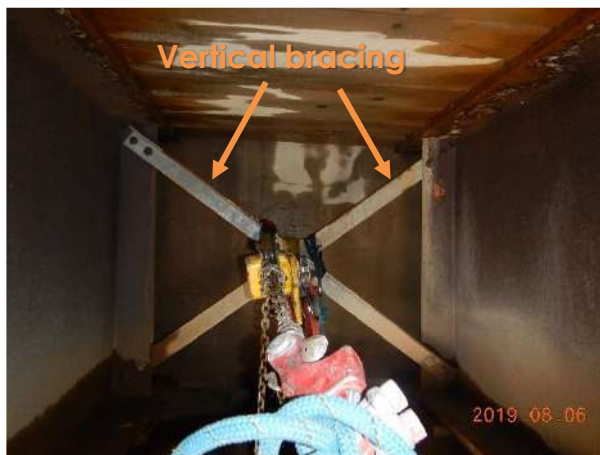
Span 1 – End vertical transverse bracings (pier 2)
