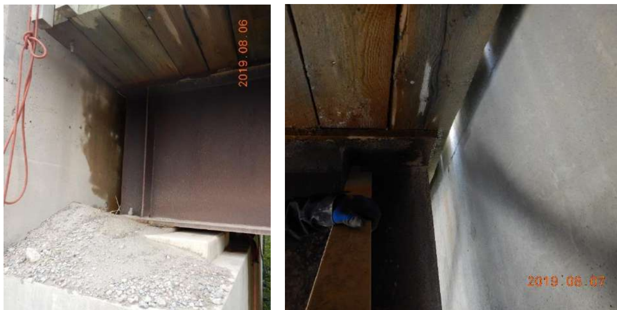
Figure 21 : Ballast walls (Left: West and Right: East)
