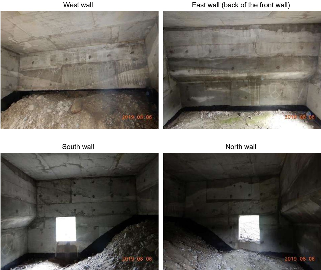
Figure 22 : West abutment's interior
