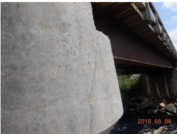
Vertical crack width < 0.8 mm
