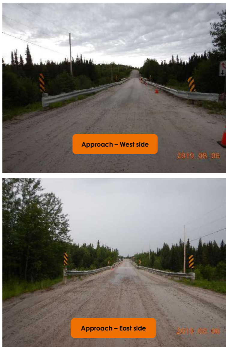
Figure 14 : Wood and galvanized steel Guardrails
