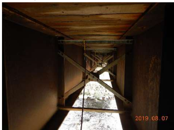
Span 2 – Timbers between beams
