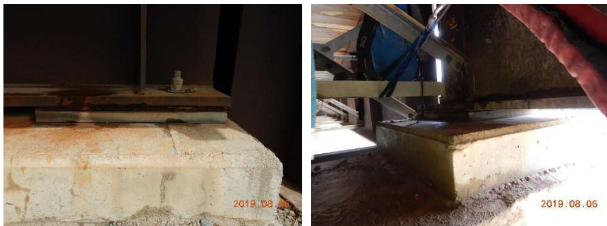
Figure 28 : Pile's bearings and pedestals
