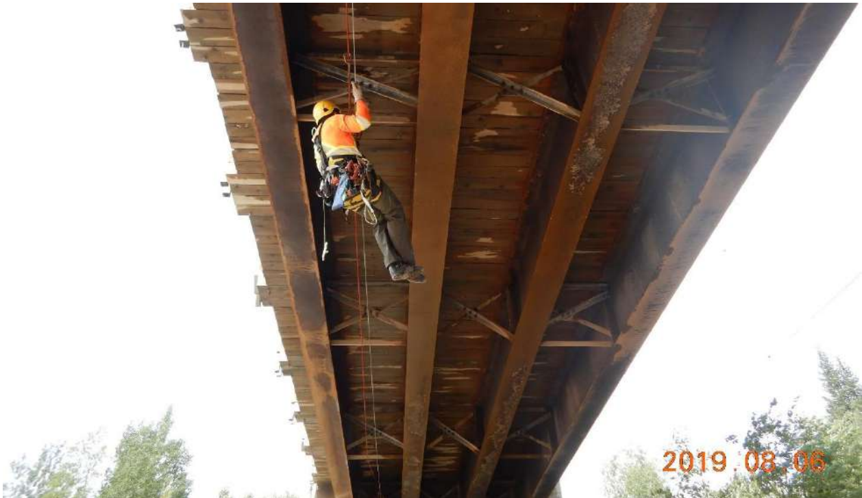
Figure 4 : Beams and wood deck
