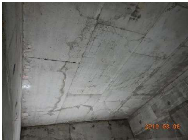
West abutment: Deck soffit
