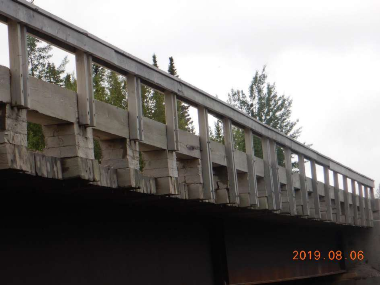
Figure 35 : Wood guardrails – span 2
