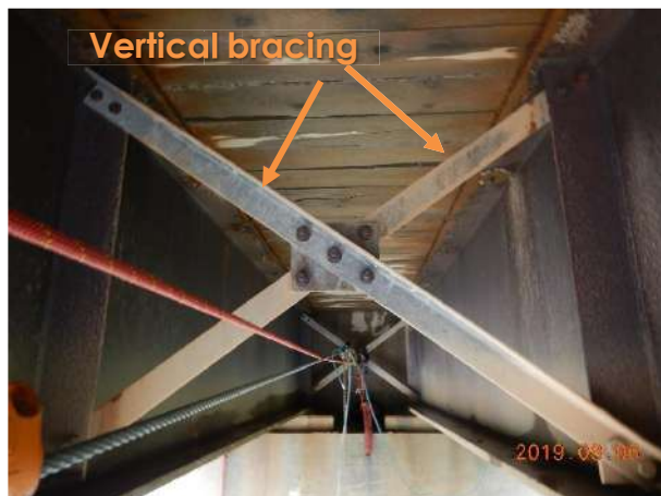
Span 2 – Intermediate vertical transverse bracings and horizontal bracings
