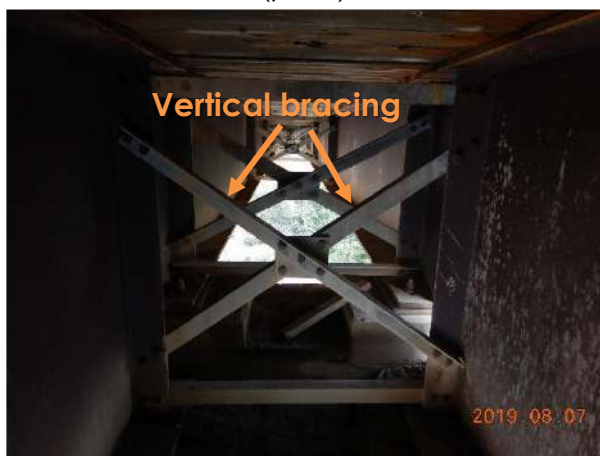
Span 1 – End vertical transverse bracings (pier 2)
