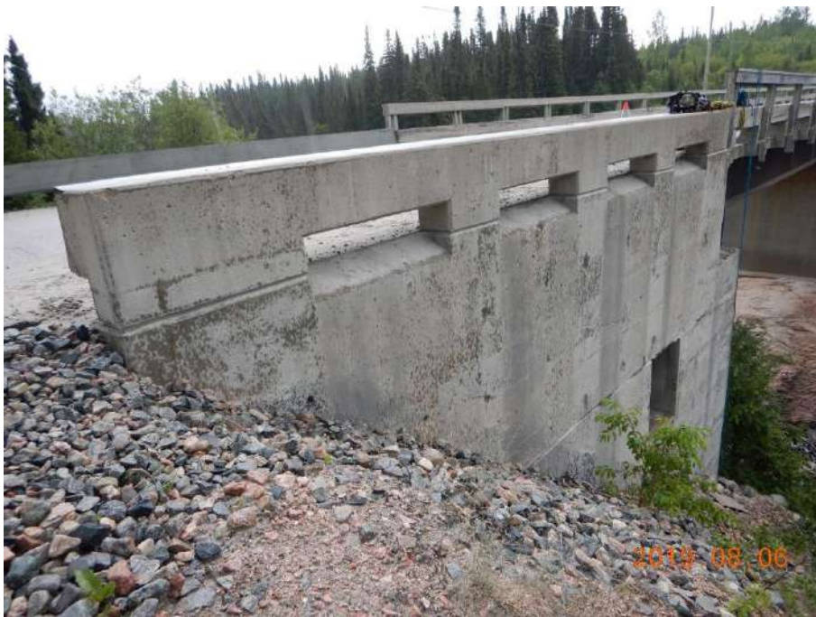
Figure 13 : Slope protection, wingwall no.1
