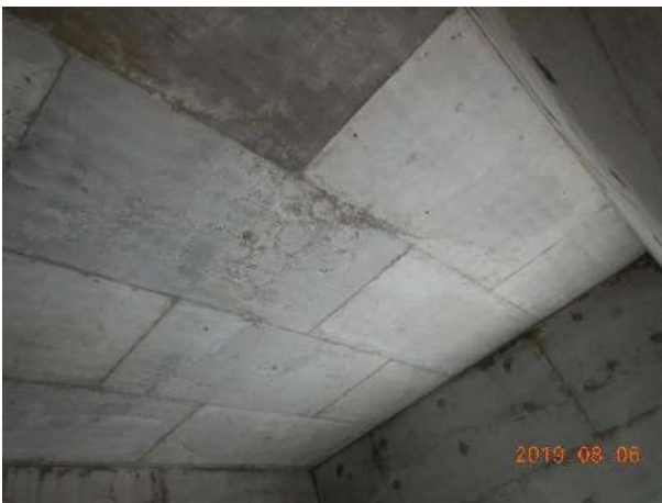
East abutment: Deck soffit
