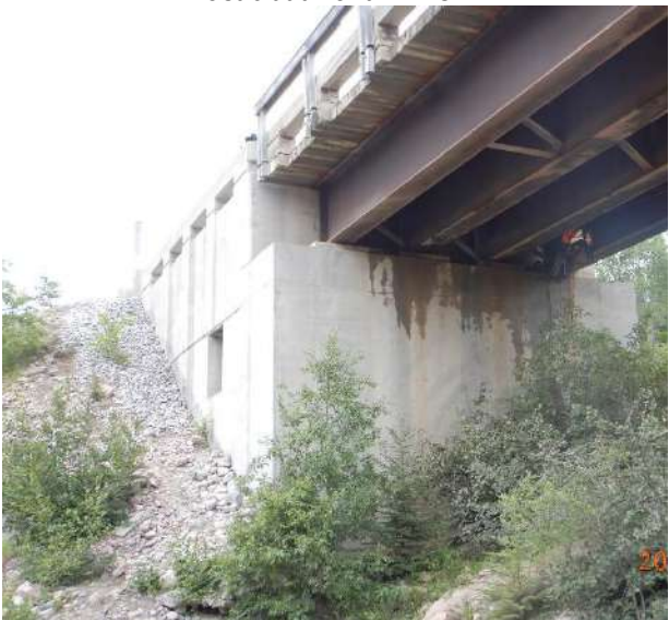
West abutment / Axis 1
