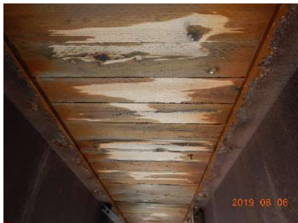
Span 1 – Timbers between beams
