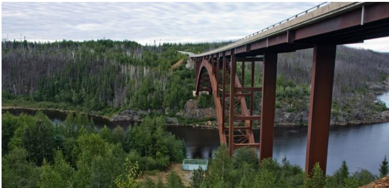
Figure 3-1 Current Roadway Bridge over Eastmain River
