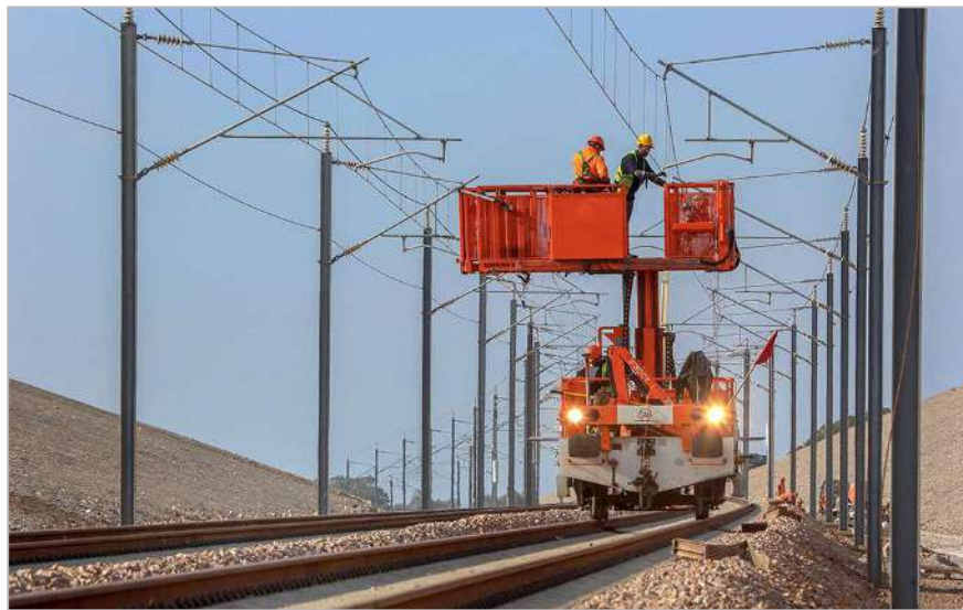
Figure 4-2: OCS 2*25 kVac type for main tracks
