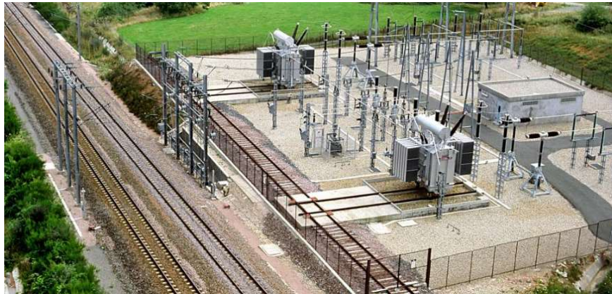
Figure 5-4: Picture of a 2*25kVca substation
